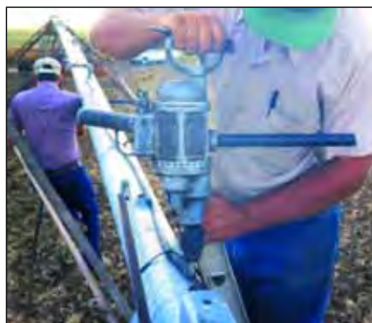
Figure 13. Drilling for swedge coupler.
