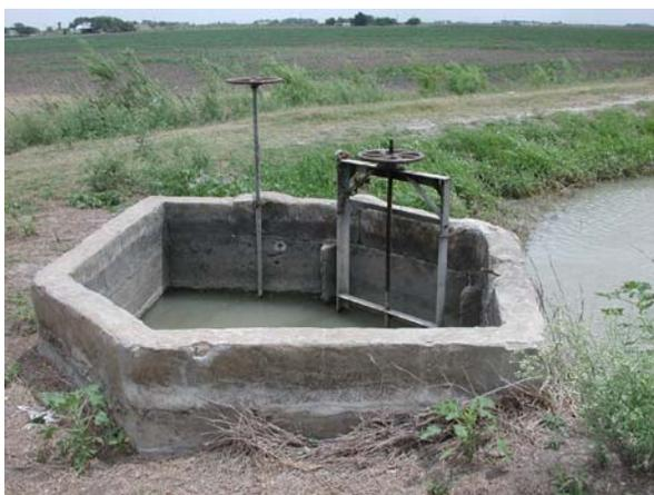
**Figure 9. A box head gate situation that typical occurs at the beginning of a canal or after a road crossing. This controls downstream, levels and supplies usually two farm turnouts.**
