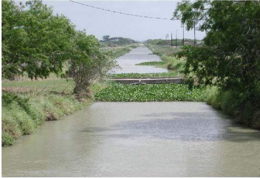
**Figure 2. Culvert clogged by aquatic vegetation (Water Hyacinth)**
