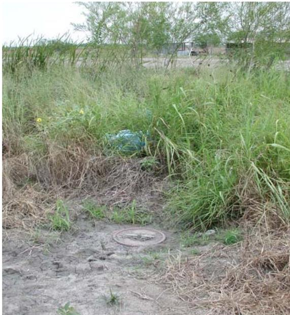
**Figure 11. Farm turnout valve at canal 27 and B.**
