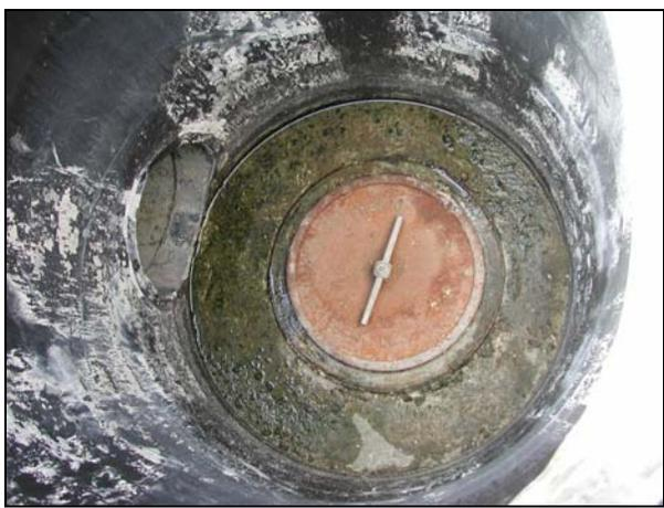
**Figure 6. Typical 14-inch *Fresno* alfalfa valve used in the district.**
