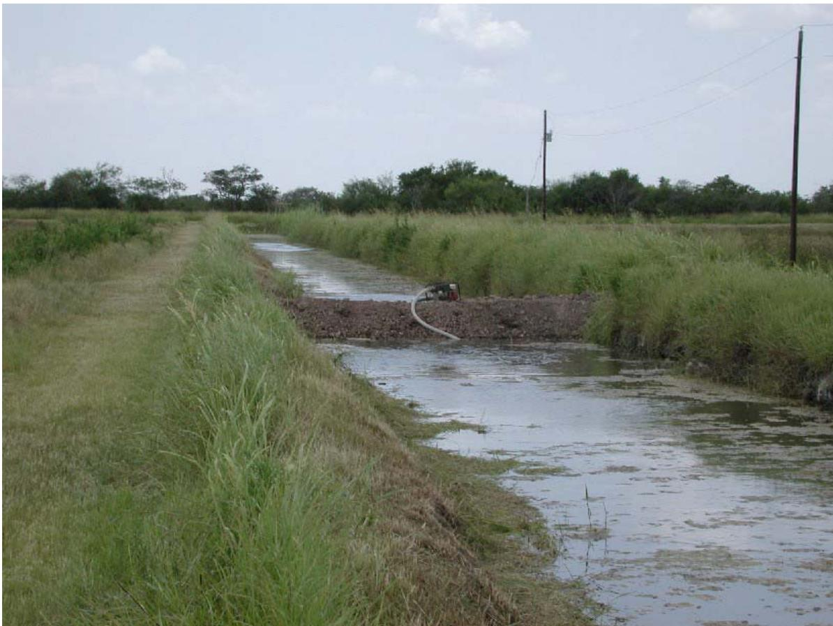
Figure 1. Earthen dam constructed on canal 55.
