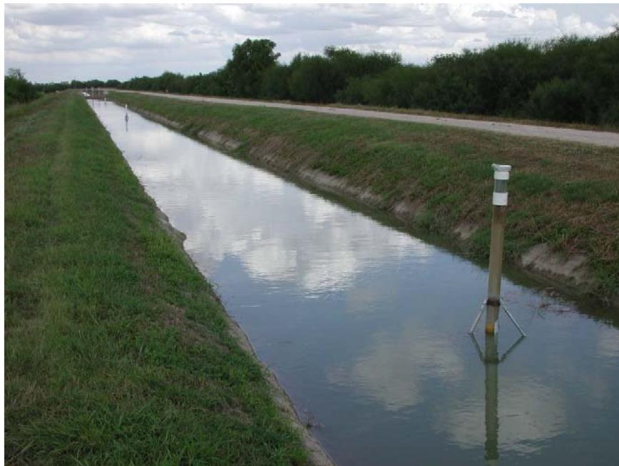
Figure 10: Continuous stage level recorders on Lateral A – “I” Rd.
