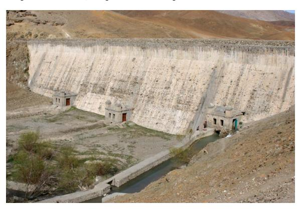
The dam has many serious problems: cracks, an eroding face with numerous holes, with one that penetrates through the dam and leaks. Nor does the dam have an emergency spillway. All which spell dome for the dam; I estimate that without repairs, the dam will collapse in two to three years.
