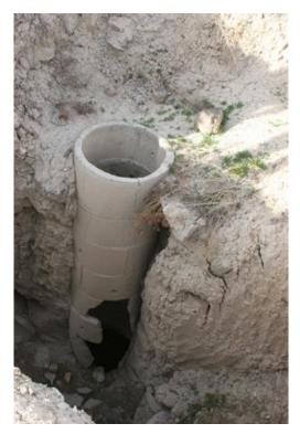
The water well in the court yard is in just as bad shape, partially collapsed as well. They have dug a deep ramp to the remaining well casing in an attempt to prevent further collapse and to provide water access.
