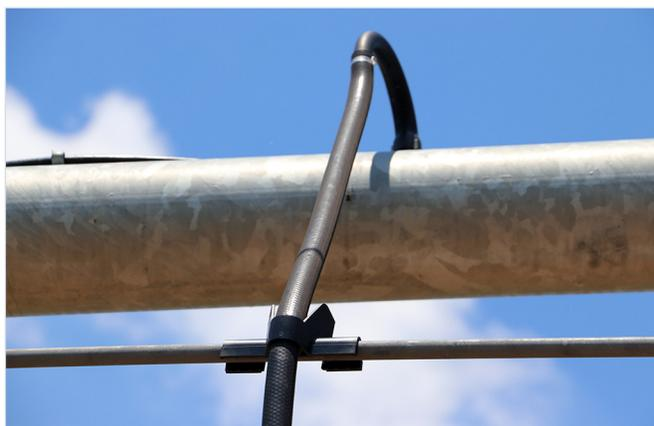
Figure 9. Truss rod hose clamps/slings.
