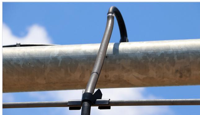
Figure 9. Truss rod hose clamps/slings.
