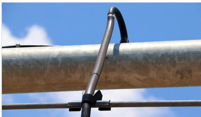
Figure 9. Truss rod hose clamps/slugs.
